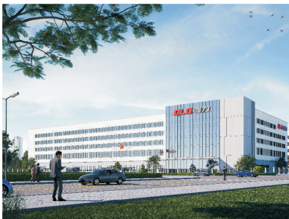
• 翁垟工业园(兴建中) Wengyang Industrial Park (Being Constructed)
